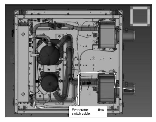
Fig. 14 – Cables routing of evaporator flow switch
